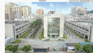
Dongguan Plant Guangdong, China
