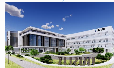
New Headquarter Taichung, Taiwan
