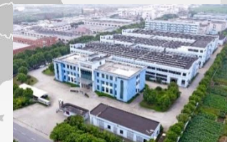
Jiashan Plant Zhejiang, China
